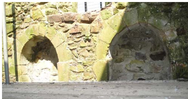
'Window' openings (D18 and D19) from interior of tower.
