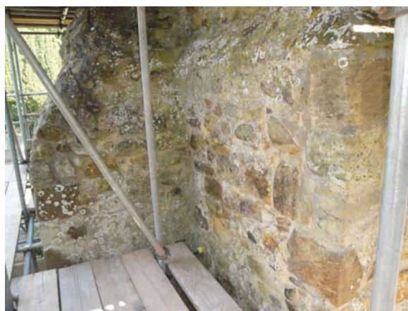
Roof of stair turret (E3).
