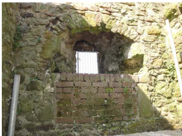
Interior of window (C5).
