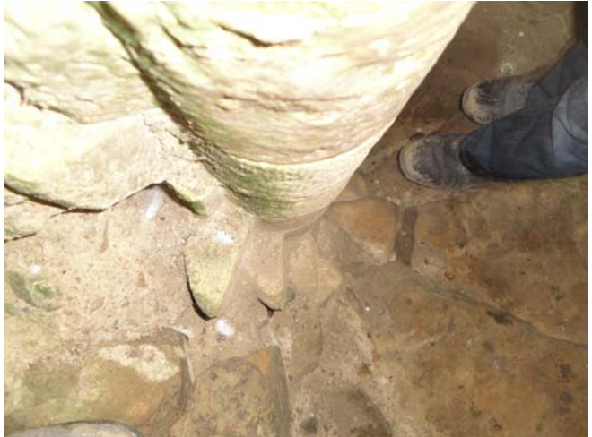
Looking down the spiral staircase (E4).
