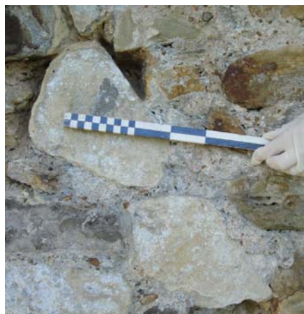
Two dressed Caen stone blocks indicating top of turret (D40).
