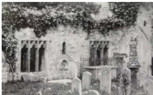
Photograph showing the north wall of the nave before windows F4 and F8 had fallen. [Photo from HAARG archive].
