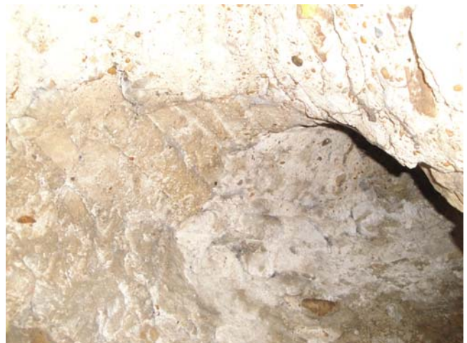
Marks of the shuttering used in the construction of the roof of the spiral staircase (E4).
