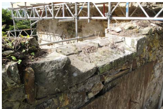
Cill of added dormer window (F5).
