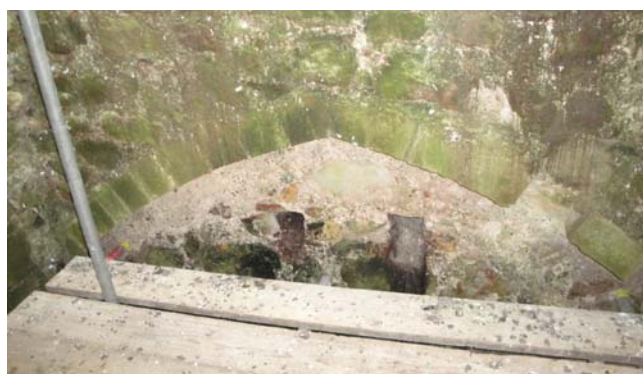
Support arch (D25) to former bell turret.
