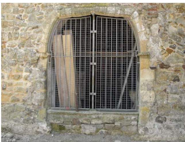
Tower arch (D5).
