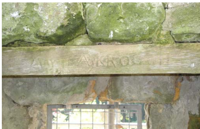
Timber lintel at head of window (B8).
