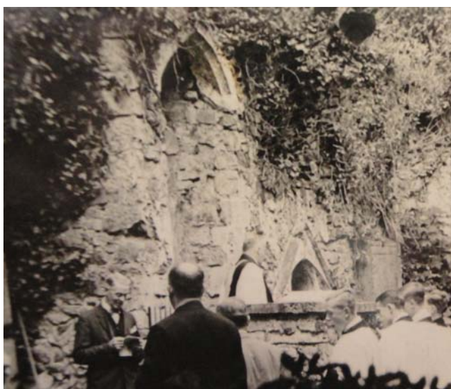
Window G2 shown prior to it having fallen. [Photograph from HAARG archives].
