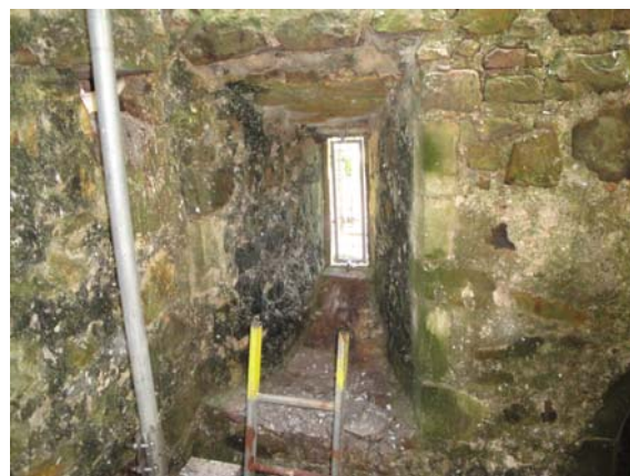
Interior of window (C3).
