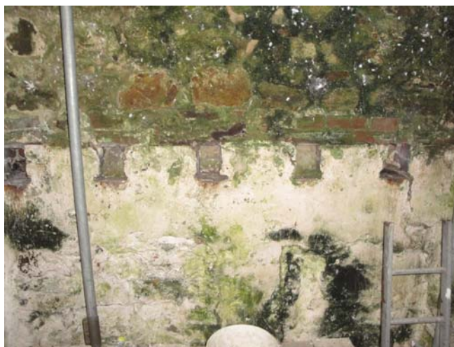
Joist sockets (A21).
