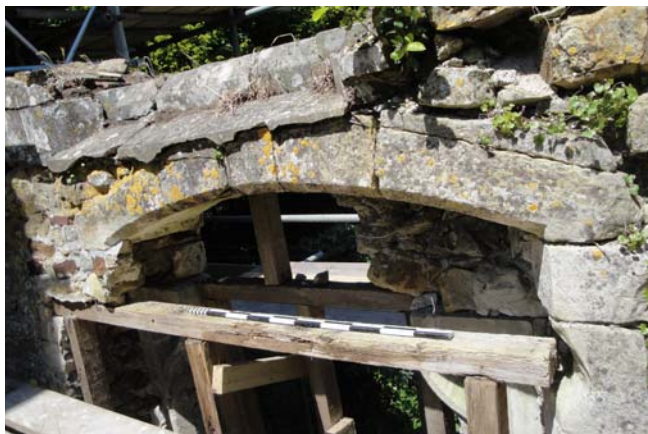
Rear arch of two-light window (F10).
