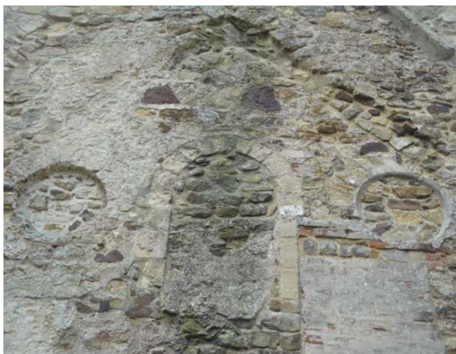
Window (D10) in the centre with circular window (D12) on left and circular window (D13) on right. Roof scar (D14/D15) is visible above the windows.
