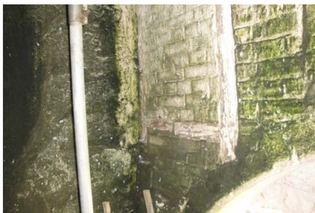
Blocked doorway (D7) leading to former gallery.
